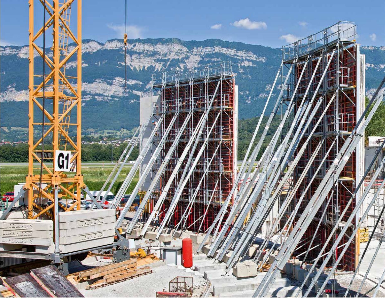
Use with VARIO GT 24 Girder Wall Formwork Bridge piers, Velim railway testing facility of the VUZ Research Institute, Czech Republic.
