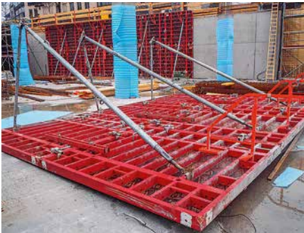
Easy and safe assembly of push-pull props and kickers on horizontally-positioned formwork, ...
