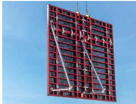
... moving the preassembled wall formwork units including push-pull props with the crane ...
