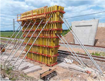
Use with VARIO GT 24 Girder Wall Formwork Bridge piers, Velim railway testing facility of the VUZ Research Institute, Czech Republic.
