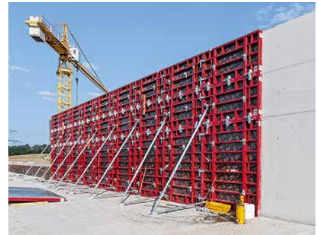
... and installation at the required position.
