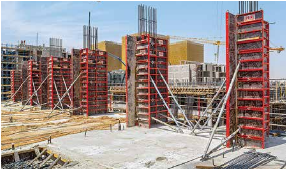
Use with LICO Column Formwork ITCC Phase II, Riyadh, Saudi Arabia.
