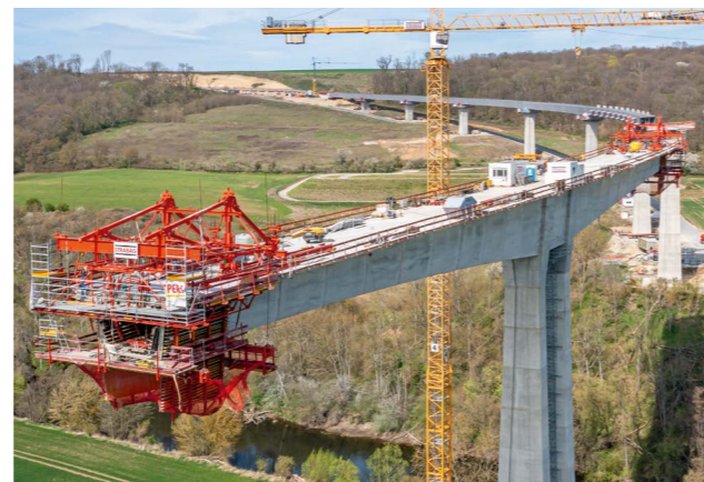
The Saaletal Bridge was built using a hybrid construction method. For the section that was implemented using the balanced cantilever construction method, the VARIOKIT VBC Balanced Cantilever Carriage was used for the first time in Germany.
