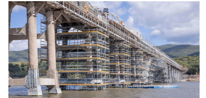
Using formwork and scaffolding systems from a single source accelerated the construction process.
