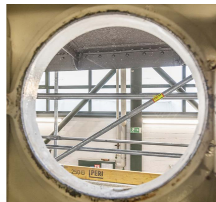
PERI delivered an efficient scaffolding solution to meet the specific requirements of this unique project.
