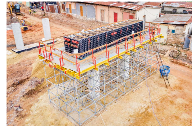
The versatility of the PERI Solution is based on the fact that a small number of components could be used for different bridge sections.
