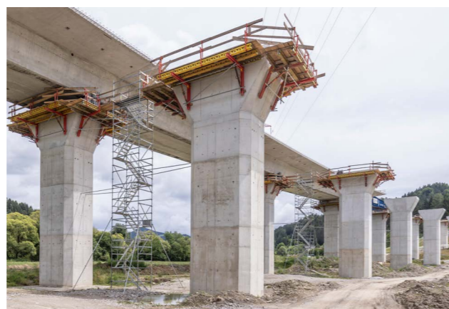
Combined with PERI UP, the flexibility of VARIOKIT made for a safe and fast construction process.
