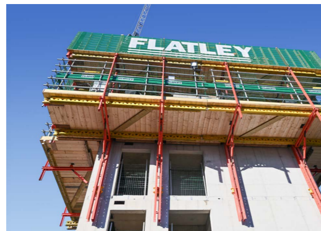
With RCS MAX Rail Climbing Formwork, all platforms could climb simultaneously. This meant that there were no gaps between the platforms, improving worker safety.
