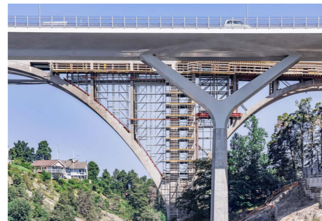
The arch of the bridge was built at a height of 32 m. PERI provided project-specific solutions and technical expertise.
