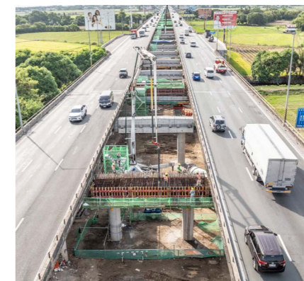
The customised PERI Solution facilitated rapid construction progress without interrupting traffic.
