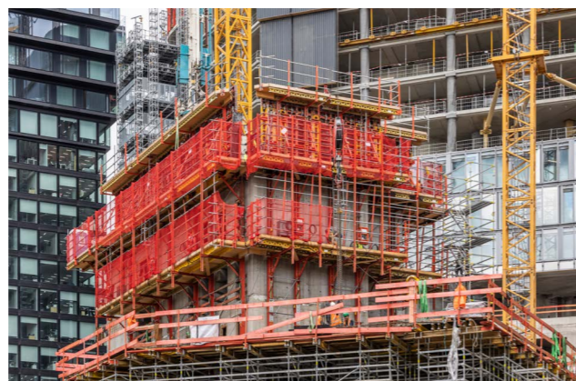
The decision to use the RCS MAX Rail Climbing System resulted in a particularly high level of efficiency and safety.
