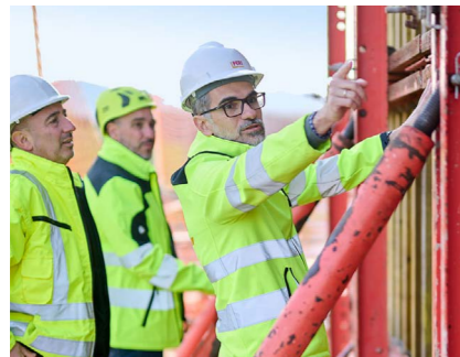
The PERI Assembly Team oversaw the on-site installation process and was on hand to answer any questions.
