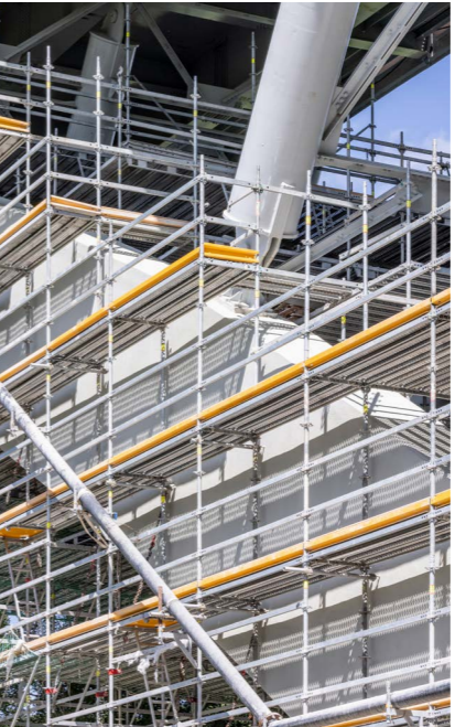
The closed deck surfaces of the PERI UP Scaffolding Kit enabled the team to work safely at height.
