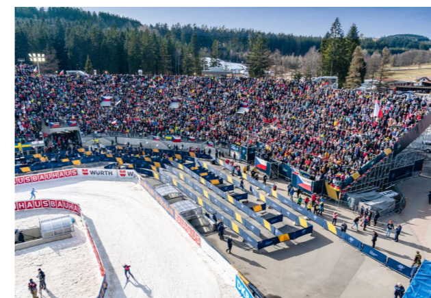
PERI UP Scaffolding and the PROKIT Lateral Protection System were used to expand the event infrastructure of the Vysočina Arena for the Biathlon World Championships.
