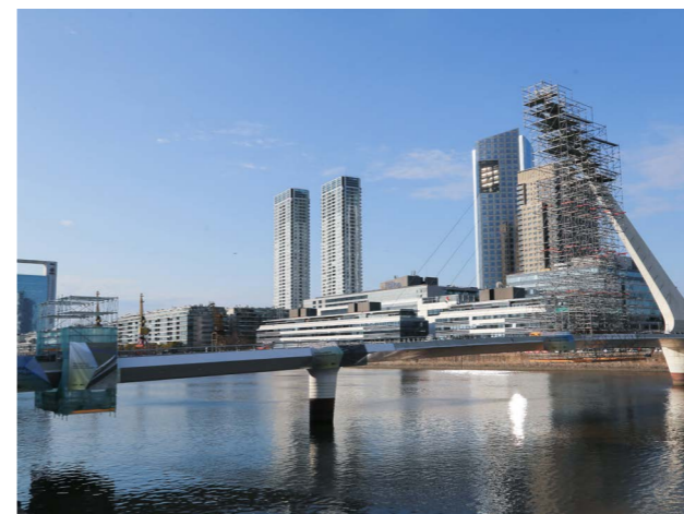
The mobile scaffolding was moved by 3 m every four days, while the sides and underside of the bridge were painted at the same time.
