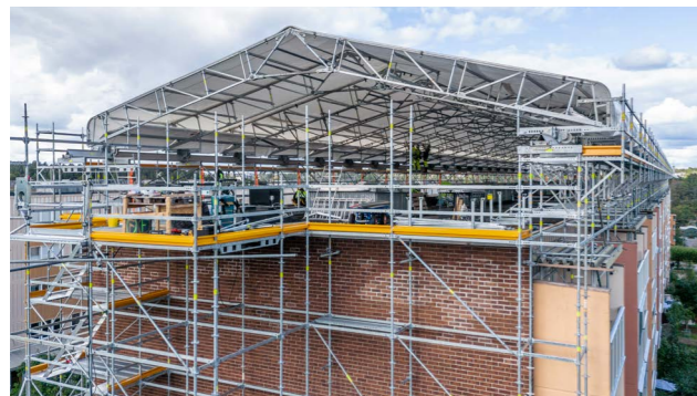
The PERI UP LGS 75 is a slender weather protection roof that was able to bridge the span width of 13 m with ease.
