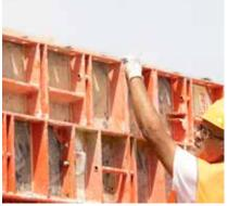
Whether during transport or assembly, thanks to the handles that are integrated into the panel, you can easily and flexibly grab the panels by hand.
