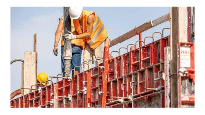
HANDSET Alpha is a robust entry-level formwork system for walls, foundations and columns. The system consists of a low number of sophisticated components and multifunctional panels that make handling intuitive.
