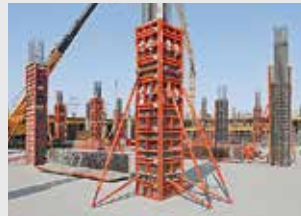
Column Formwork
