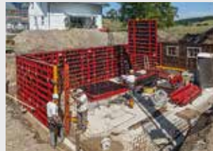
Wall Formwork
