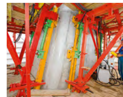
With the help of the central power supply unit, the eight hydraulic ACS climbing devices were able to climb in perfect synchronization.
