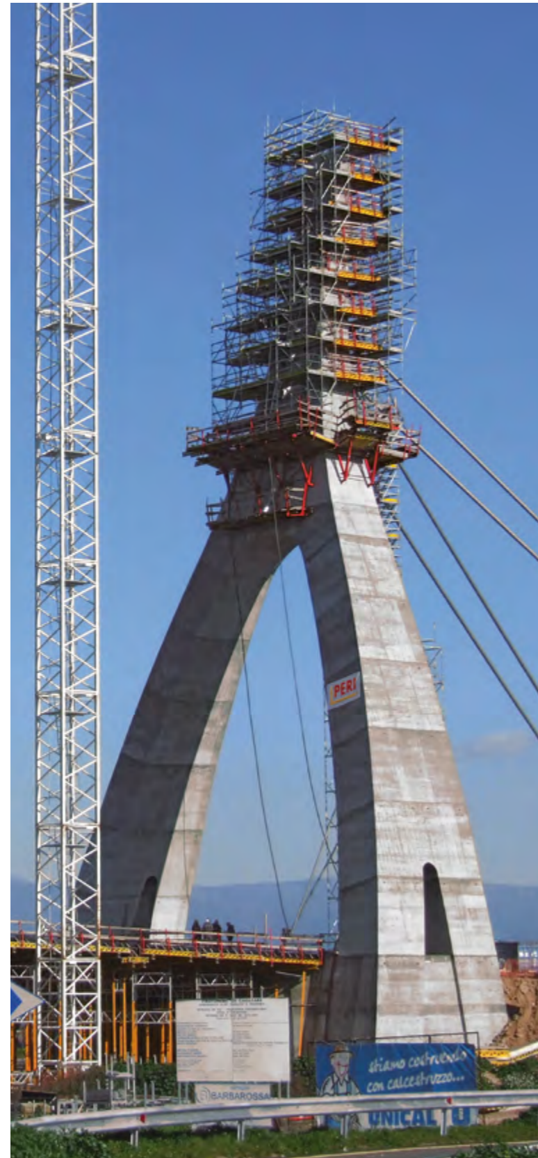
Stair access to the PERI UP working scaffold, which nestled up close to the tip of the pylon thus ensuring safe assembly of the cable-stays.
