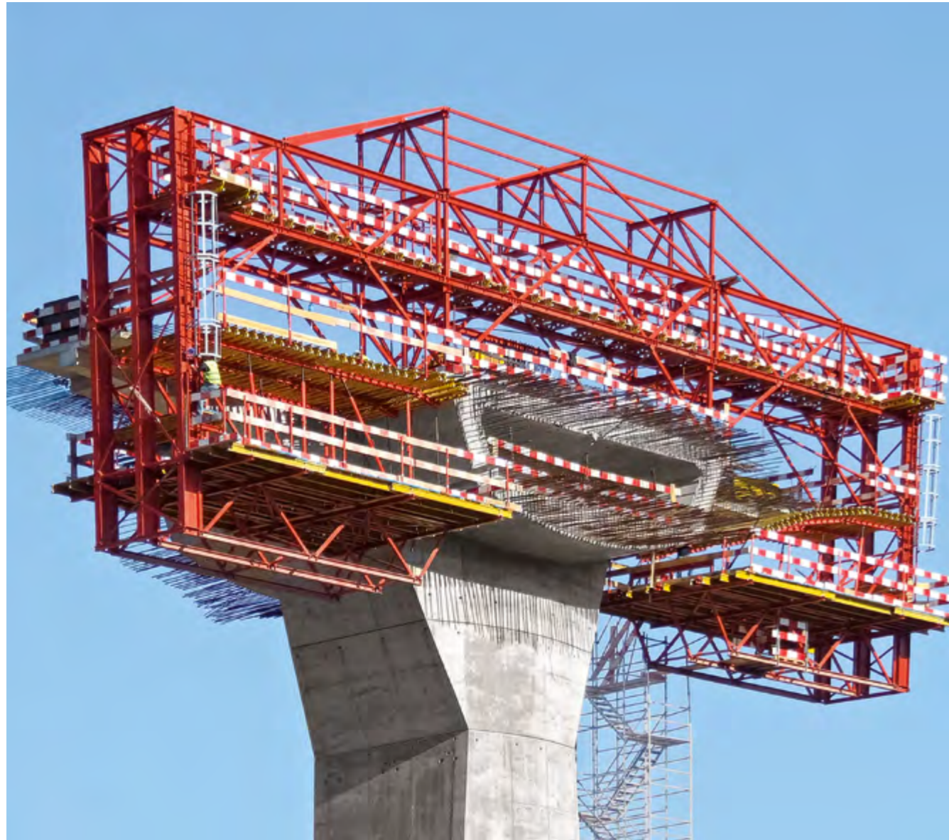
The 8 m carriageway slab was constructed in the area of the pier heads in three sections each with a 3.50 m cycle length.
