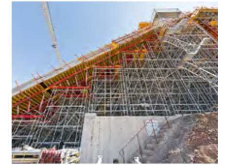
PERI engineers combined two modular construction systems to form a comprehensive load-bearing concept with heights of up to 20 m.
