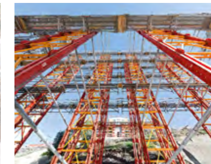
Up to 28 m high VARIOKIT heavy-duty shoring towers, combined with PERI UP, supported the bridge superstructure in the edge sections.
