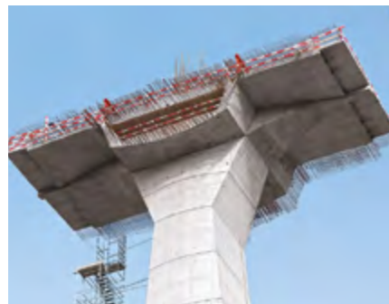
The 8 m carriageway slab was constructed in the area of the pier heads in three sections each with a 3.50 m cycle length.
