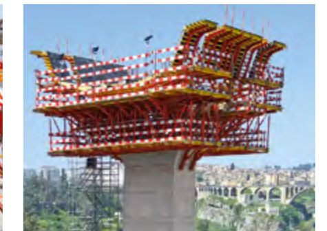
For the slab and web formwork of the starter, PERI engineers combined horizontally-positioned brace frames with VARIOKIT frame construction units.
