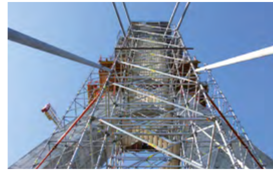
Stair access to the PERI UP working scaffold, which nestled up close to the tip of the pylon thus ensuring safe assembly of the cable-stays.
